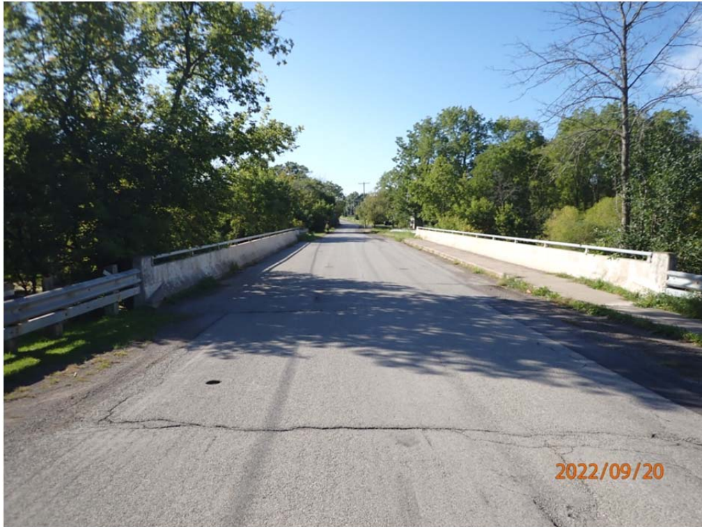
Photo No. 1: Roadway over the structure looking south.
