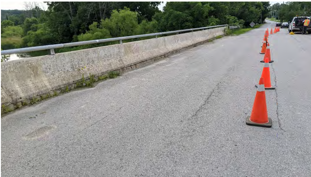
Figure F-2b Overview of bridge deck facing south.
