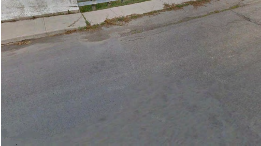
Figure F-3a Overview of paved joint at north abutment facing west.
