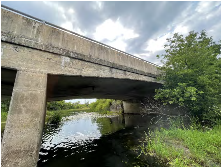
Figure F-1b Overview of west elevation facing east.
