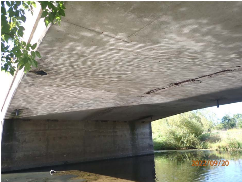
Photo No. 2: Roadway and barrier wall over the structure.
