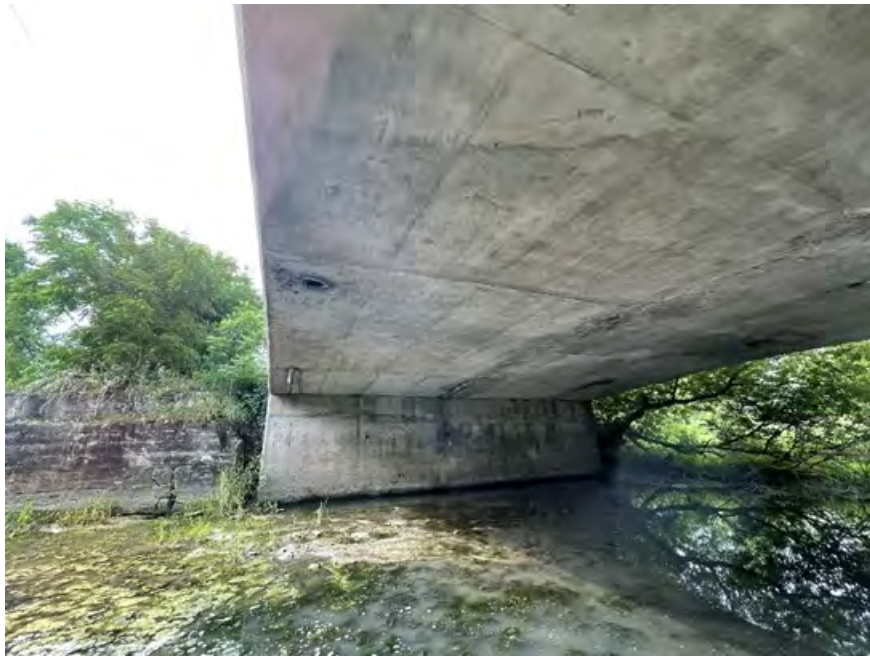
Figure F-9a General overview of south abutment facing southwest.
