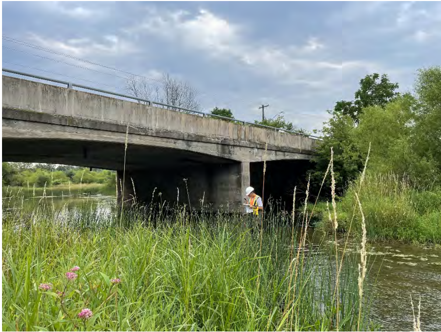
Figure F-1a Overview of the east elevation facing west.
