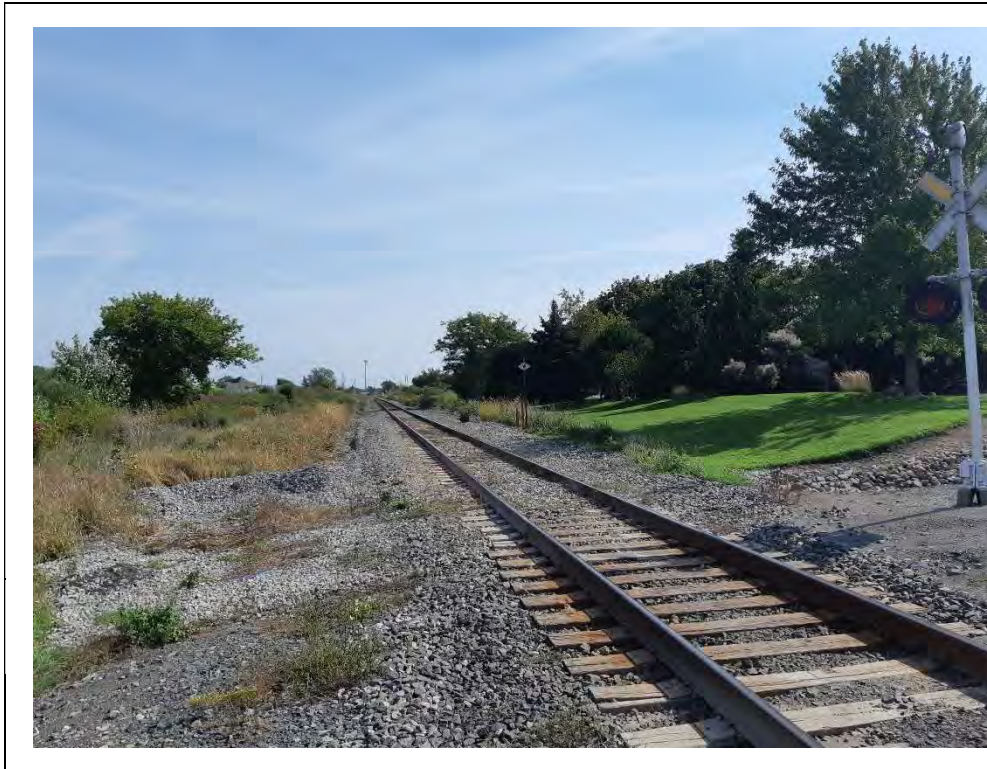
Photo 7: CP rail line, east side of Project Area.
