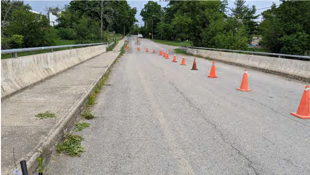
Figure F-2a Overview of bridge deck facing north.
