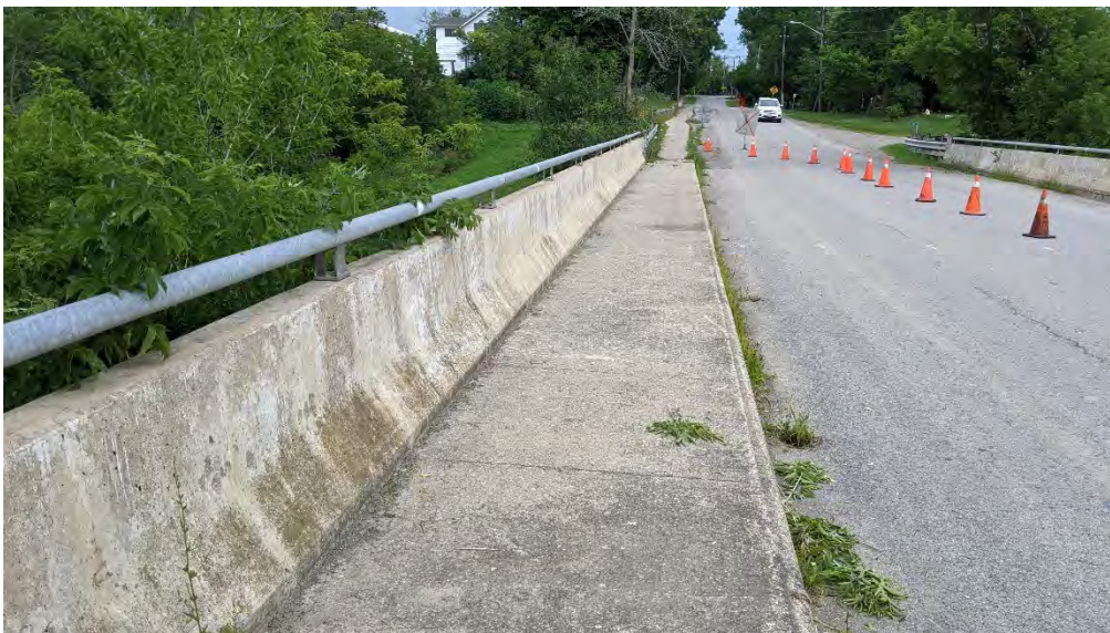
Figure F-5b Close up of west sidewalk and guardrail facing north.
