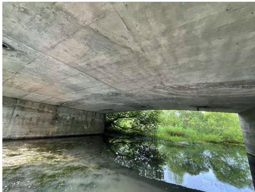
Figure F-12b General overview of south span soffit facing west.
