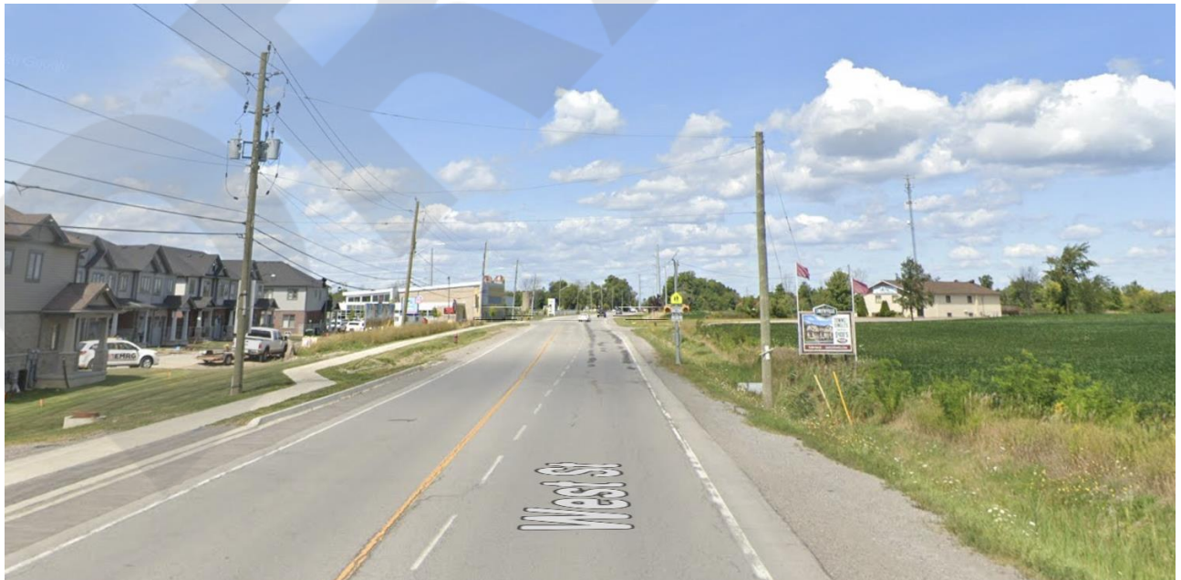
Regional Road 20 View to West
